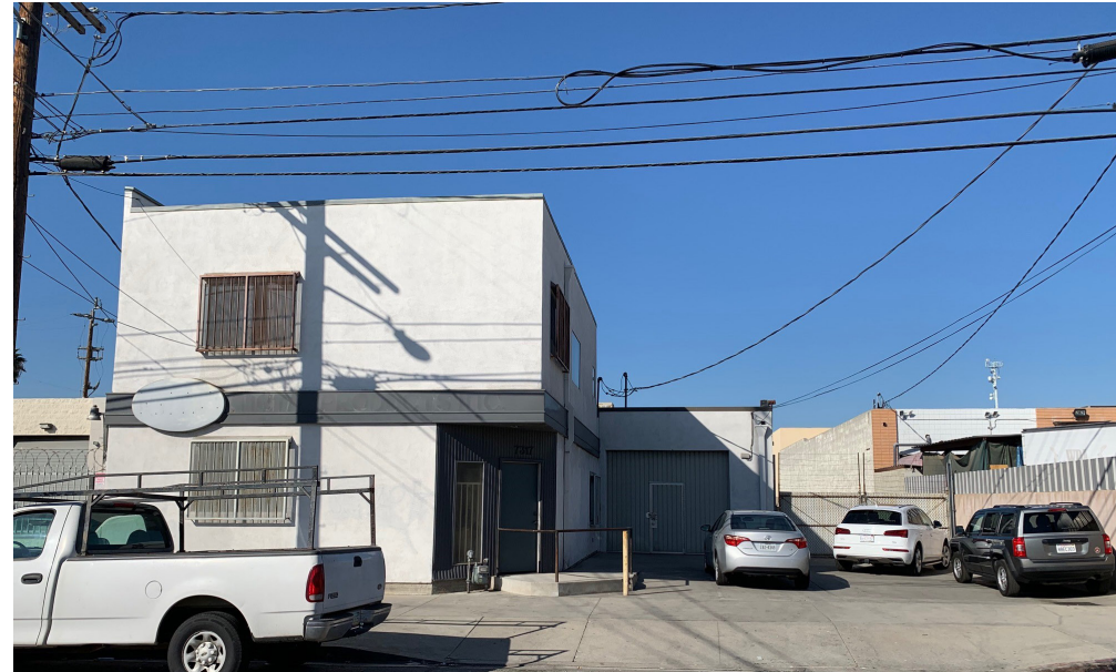
7317 Ethel Ave, North Hollywood | $2,195,000 7,300 SF Building / 16,000 SF Lot / M2 Zoning
